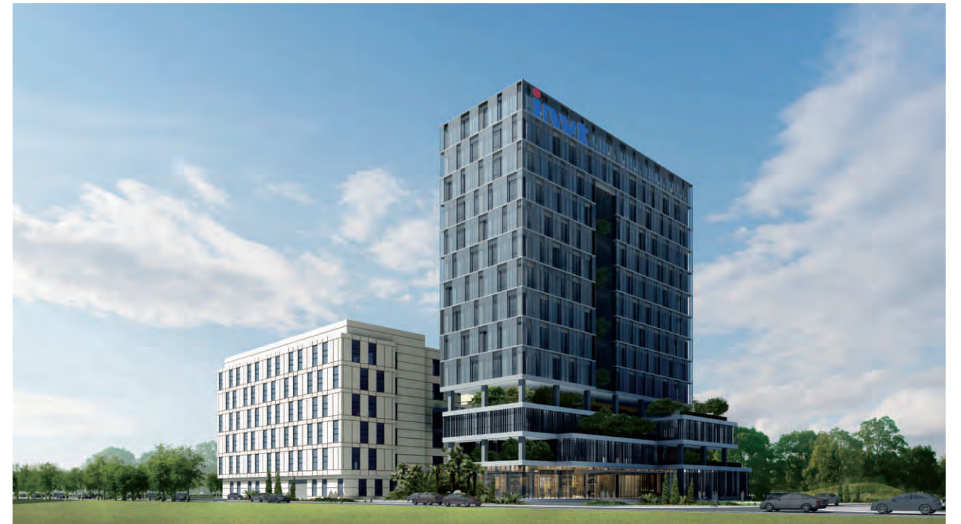
Shenzhen Industrial park
